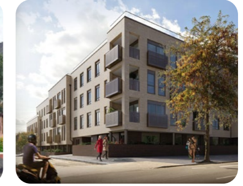
Tallack Road, Waltham Forest, London Large-scale communal Air Source Heat Pump to feed ambient temperature heat network
