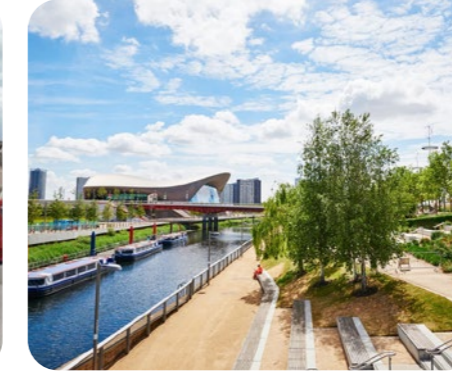
London Olympic Park, London A waste target of 90% diversion from landfill of demolition waste by weight
