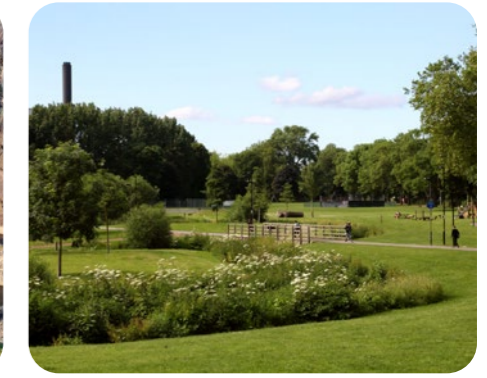
Ladywell Fields, Lewisham | SuDS Creating sustainable drainage and reduce flooding by modifying the river channel with a naturalistic setting incorporating backwaters and wetlands.
